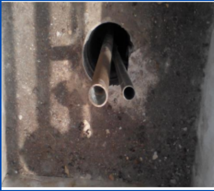
Revamped deepwell groundbed for NPDC/ Heritage Energy Operational Services Warri, Delta State Operator of OML 30
