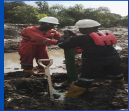
Installation of cathodic protection monitoring tetstposts on the swamp section.
